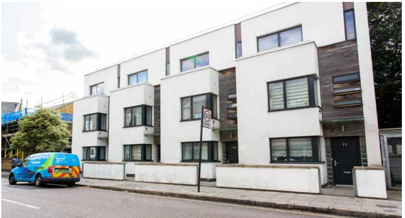
Figure 18. Boleyn Road, houses built with heat pumps
