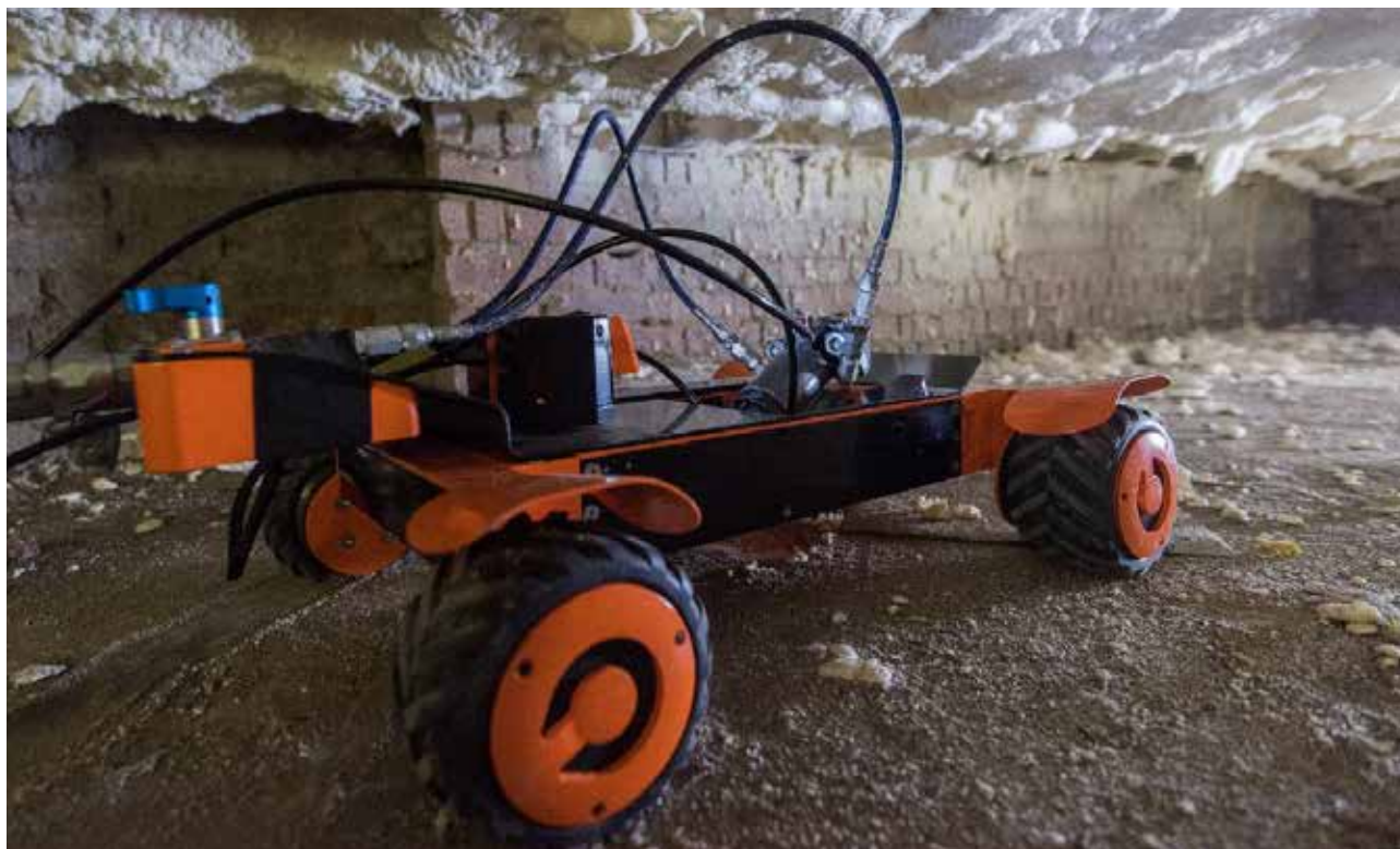
Figure 17. Installing underfloor insulation using Q-bot
