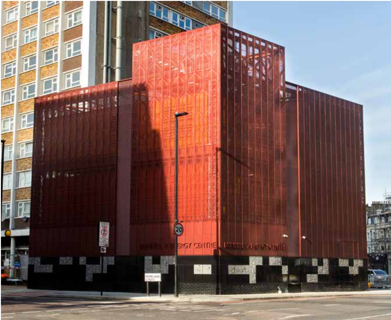
Figure 22. The Bunhill 2 Energy Centre on Central Street, which captures heat from the London Underground
