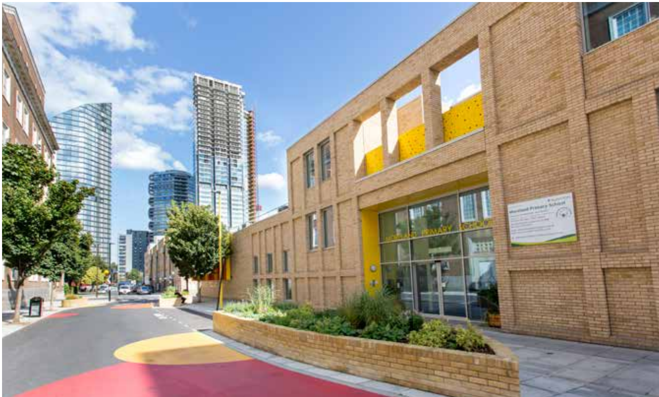
Figure 24. Moreland Primary School, one of the buildings connected to the extended Bunhill Heat and Power Network as part of the phase II project
