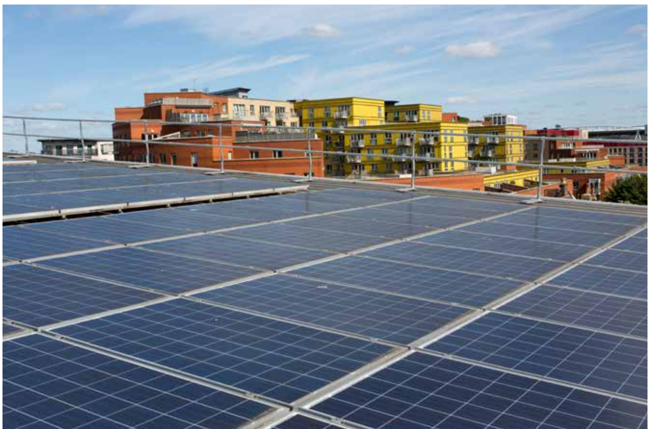
Figure 21. Solar panels on the Waste Recycling Centre
