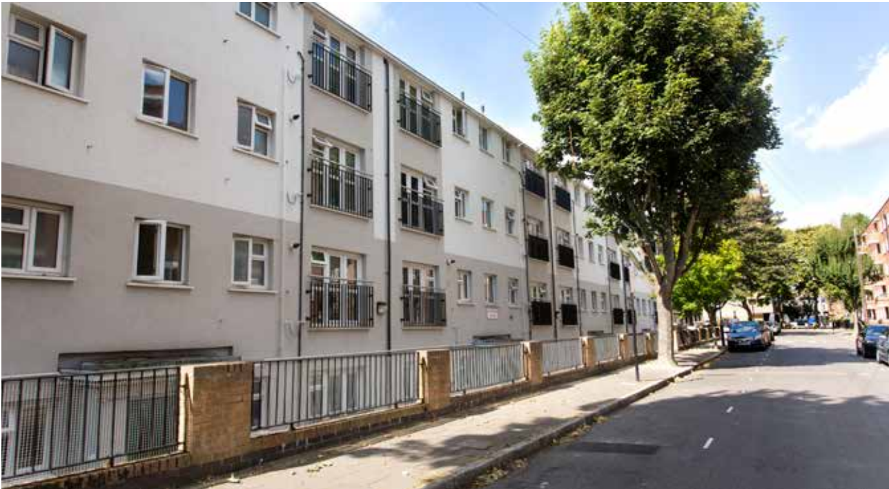
Figure 2. Solid wall insulation on Neptune House
