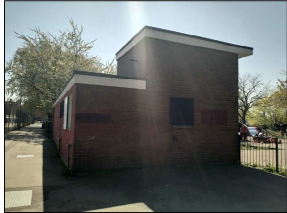
Photo 2 – Playground building (B1) viewed from the north.
