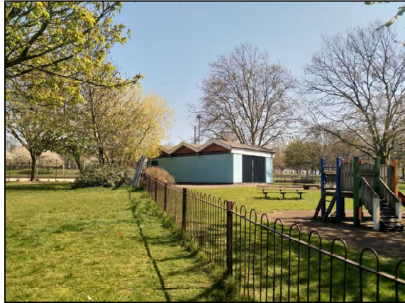
Photo 1 – On-o-clock (B2) building viewed from the north.
