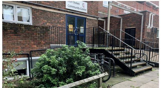
Jean Stokes Community Centre - main entrance
