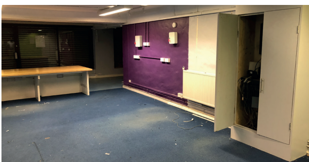
Basement space at Jean Stokes Community Centre
